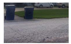
Rose Lane between Tulip Court and Aster Court, shown above, is an example of a road that is considered structurally deficient due to the road having over 25 percent alligator cracking. See the Transportation Element in Appendix A for a map displaying the Town's PASER assessment.
