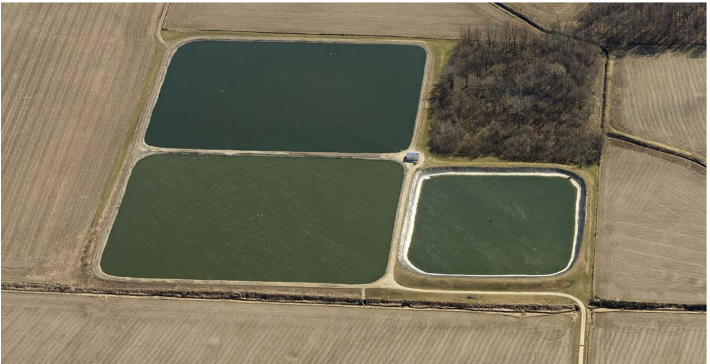
Town of Bourbon's Wastewater Lagoon System
