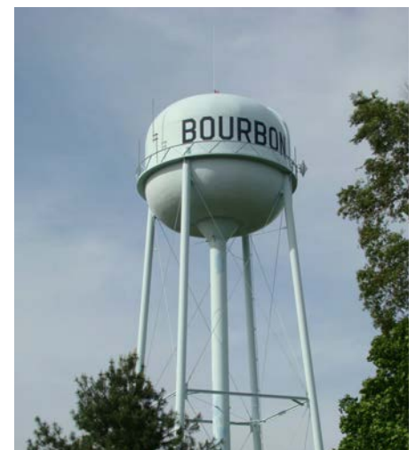
200K gallon water tank located next to corner of Thompson Street and Pine Street.
